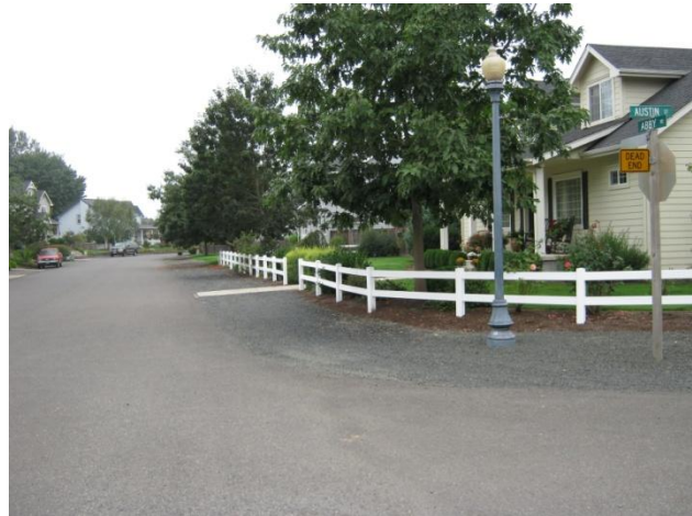
Figure 18 Existing Residential Streets
