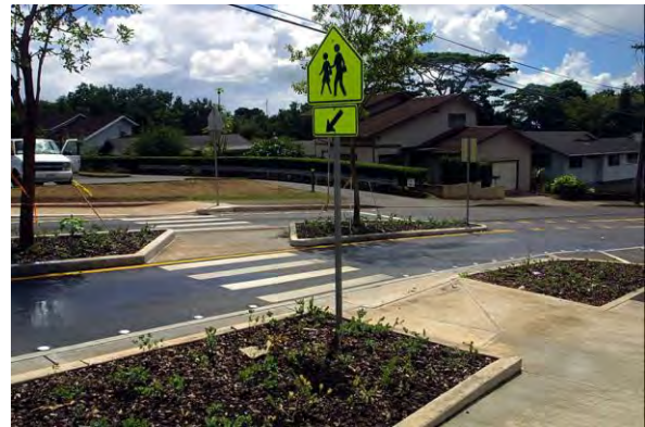
Midblock crossing assist pedestrian in safely crossing roads. All intersections contain crosswalks, whether they are marked or not.
