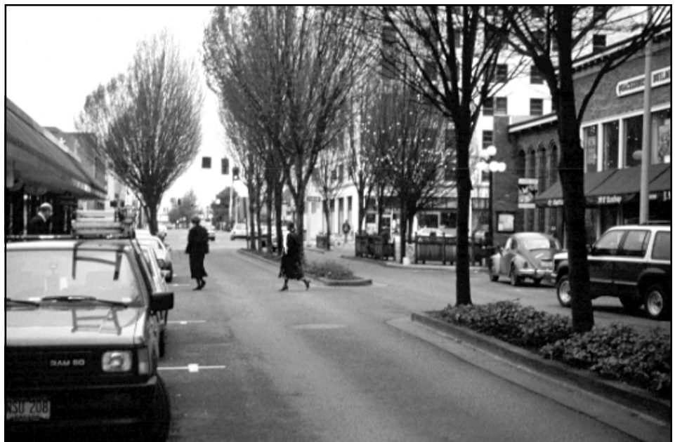
A narrow median, curb extensions, and recessed parking calm traffic on E. Broadway, a downtown collector street
