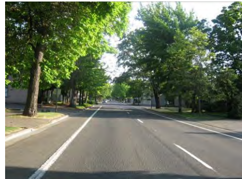
Pearl Street at 16 th Avenue is a minor arterial and contains two 12 foot travel lanes, and 5 foot bicycle lanes on both sides of the road.
