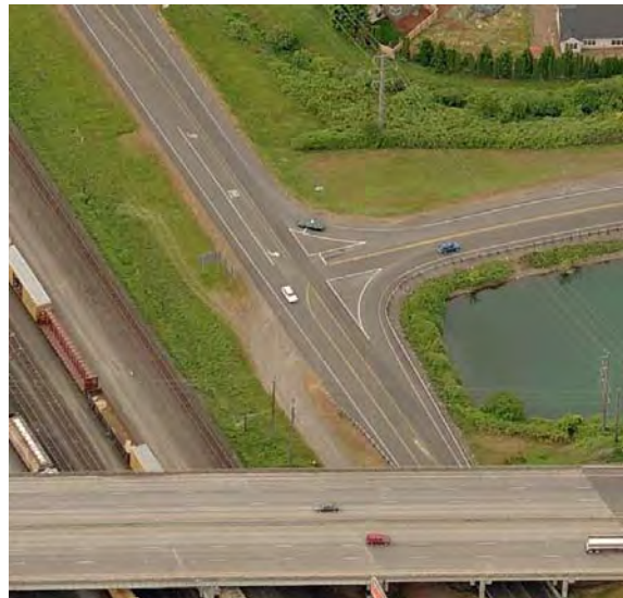
Aerial view of the Randy Papé Beltline Westbound Ramp intersection with Northwest Expressway.
