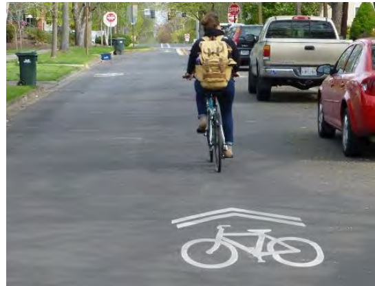
Shared roadways are one type of facility that serve both cyclists and drivers.
