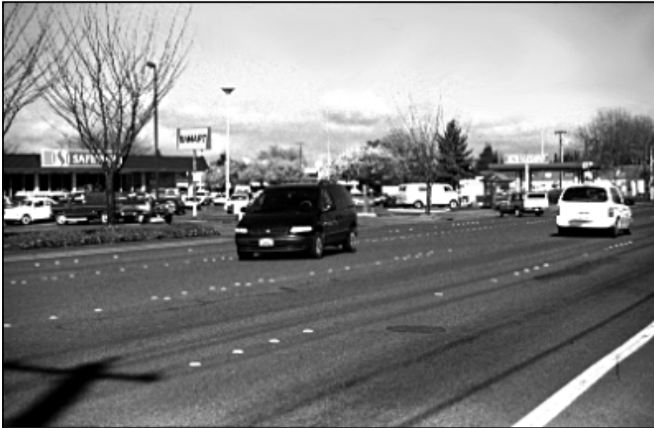
A center turn lane on River Road
