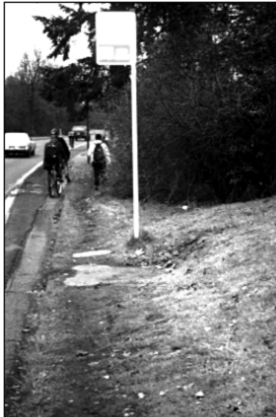
Missing sidewalk segment makes access to transit difficult
