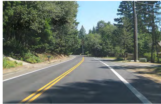
Many roads in Eugene's South Hills lack sidewalks on one or both sides.
