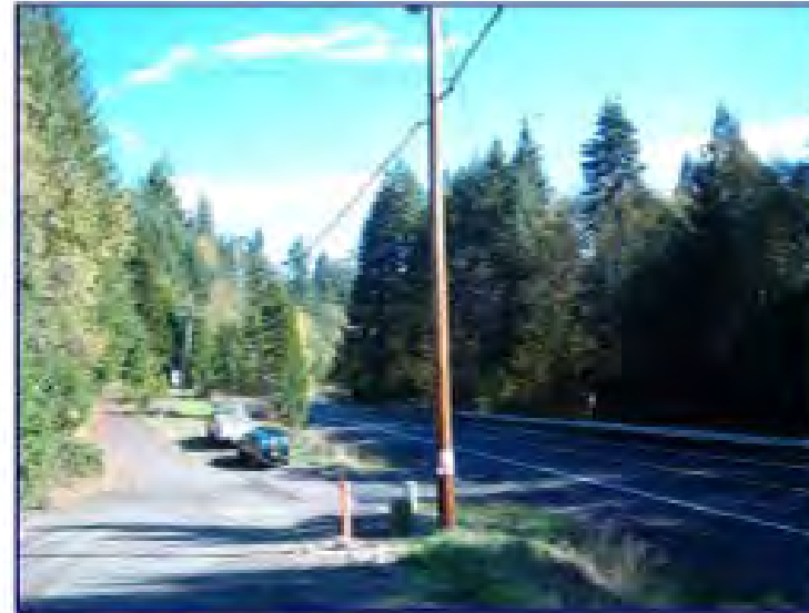
Right: Main power transmission line along Hwy. 126 and connection to underground (distant pole).
